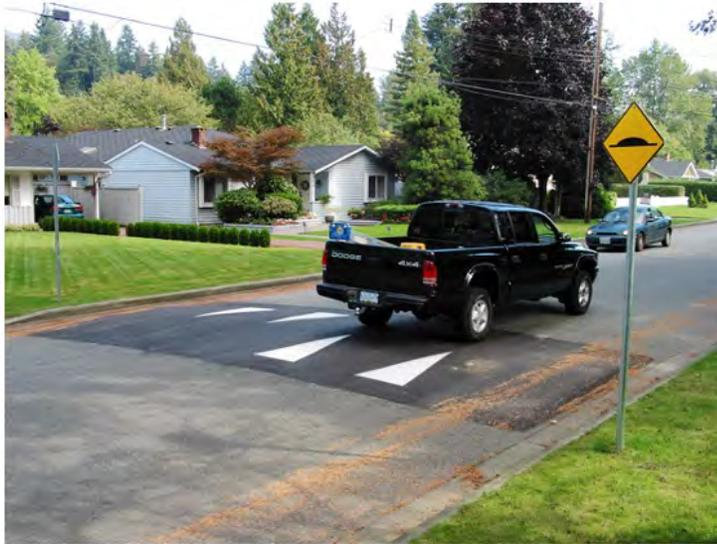
Speed humps reduce 85<sup>th</sup> percentile traffic speeds by 6 to 13 km/h
